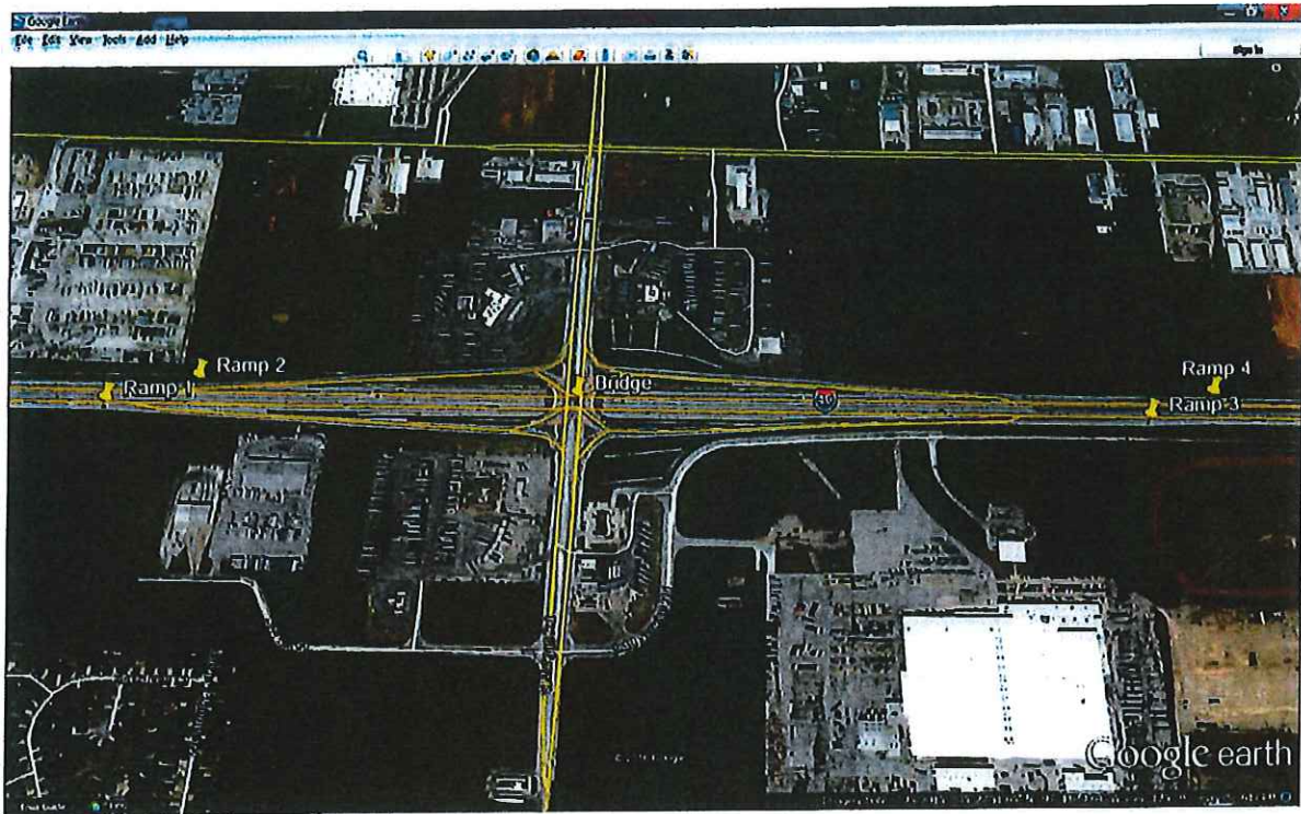
I-40 and Morgan Road Interchange (Ramps and Bridge)
